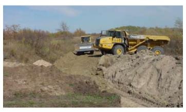
Construction of the ridge dike. Trench is dug, backfilled with clay, and compacted to prevent seepage.
