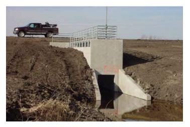
$Completed\ outlet\ structure\ /\ control\ gate.$
