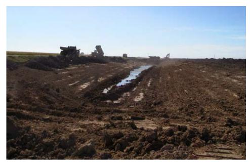
Inlet channel construction and placement of topsoil for seeding.
